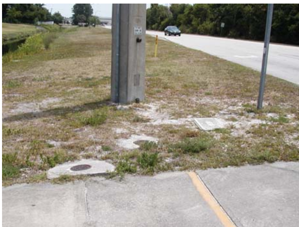
Access to pedestrian push button is not paved
