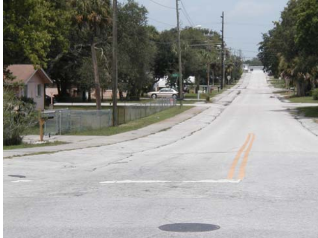
Some buffer areas between the sidewalk and roadway have been paved to reduce maintenance
